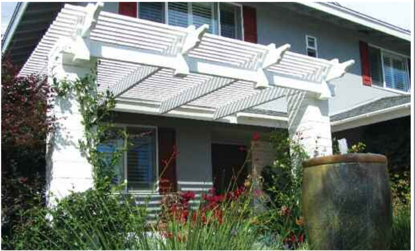
Palomar patio cover installed on brick pillars.
