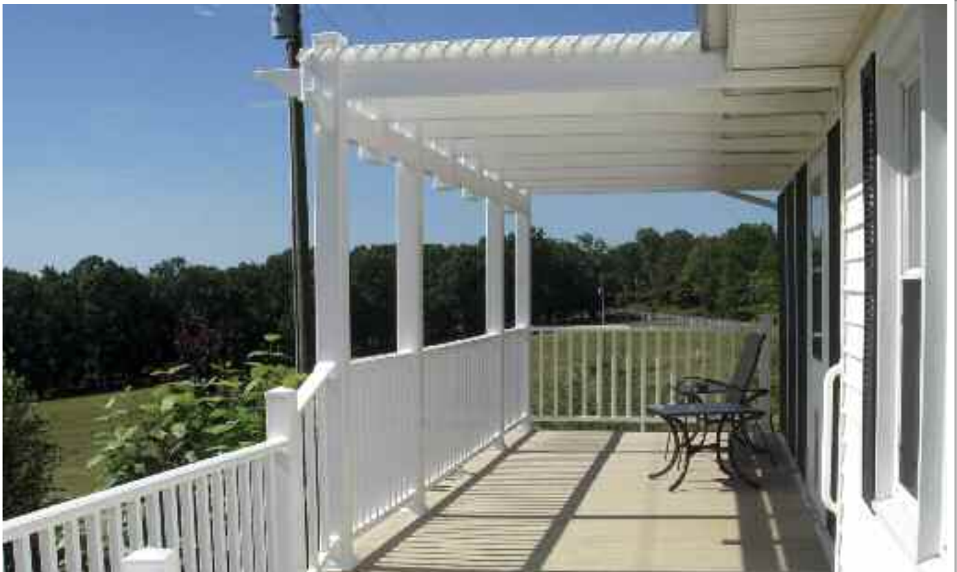
Palomar patio cover installed with railing.
